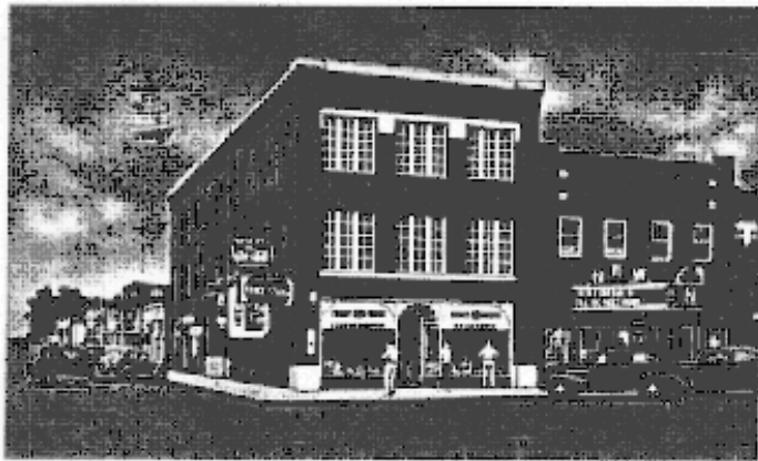
ABERDEEN, MD., CORNER BAL AIR AVE. AND PHILADELPHIA BOULEVARD 24-4831
